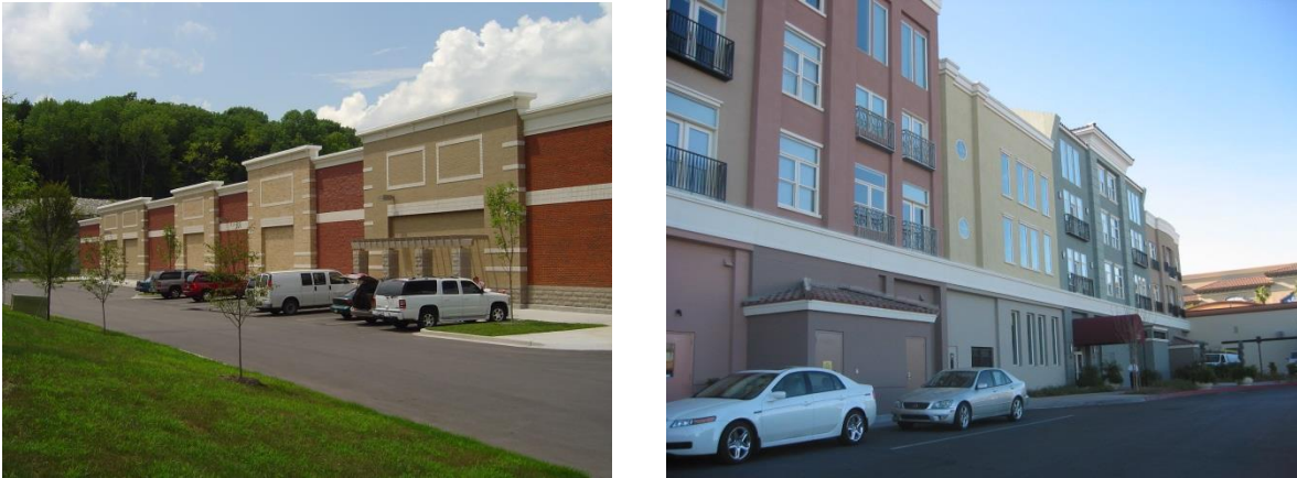
Figure 905-A: This figure shows two methods of using architectural features to create wall surface relief on wall elevations that are not the primary elevation.
