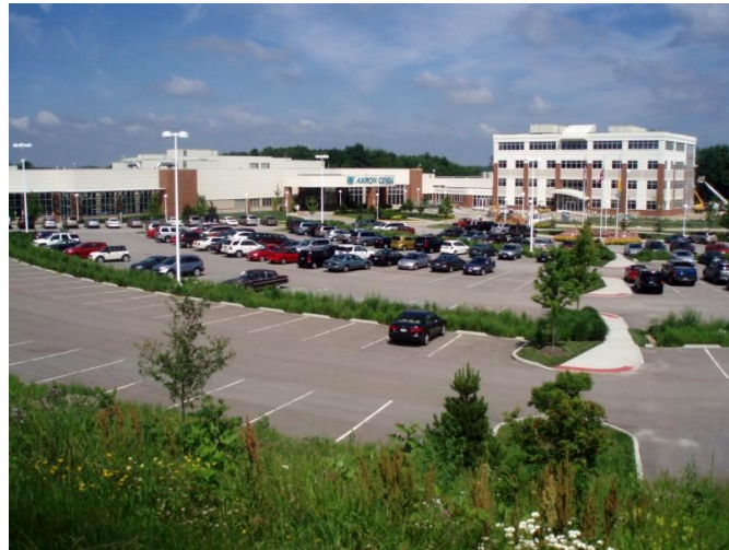
Figure 1003-A: The above image illustrates the use of natural landscaping within a vehicular use area.
