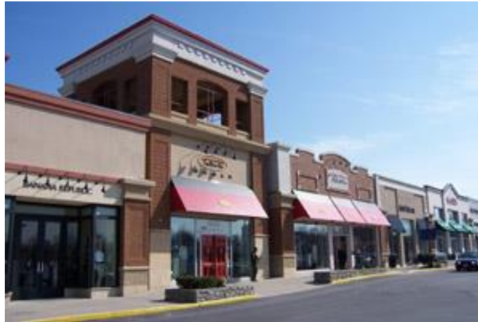
Figure 905-C: The above image illustrates a building that contains pilasters, cornices, and a series of façade setbacks (recesses) to visually break up the appearance of the large facade.
